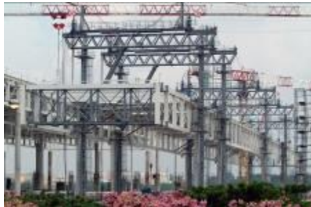
Changi Airport Terminal 3: Main pavilion roof structure
