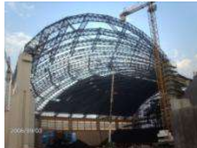
Petrochemical and Power Generation
