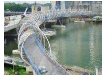
Helix Bridge: Duplex stainless steel helix framed structure
