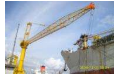
Lion Crane 1& 2: Two dock cranes at Sembawang Shipyard
