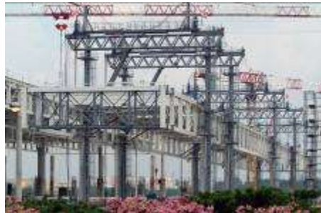
Changi Airport Terminal 3: Main pavilion roof structure
