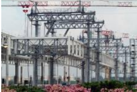
Changi Airport Terminal 3: Main pavilion roof structure
